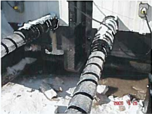
Figure 1 Wash water from washing machines in trailer from camp leaking out onto ice pad.
