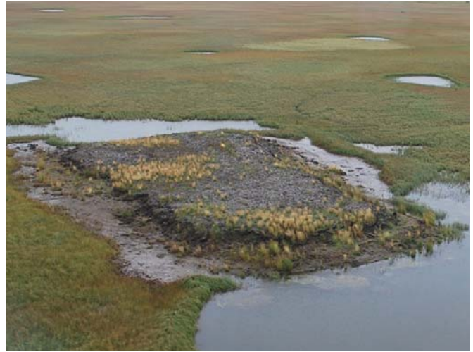
Figure 2 North end of drilling sump. Erosion occurring with sump cap edges, August 23, 2010.
