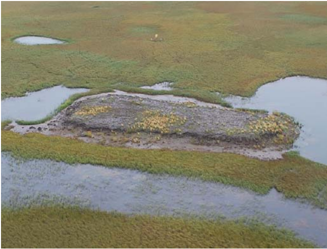
Figure 1 Kurk M-15 drilling sump. Eastern side of sump with ponding surrounding the sump and poor vegetation cover, August 23, 2010.
