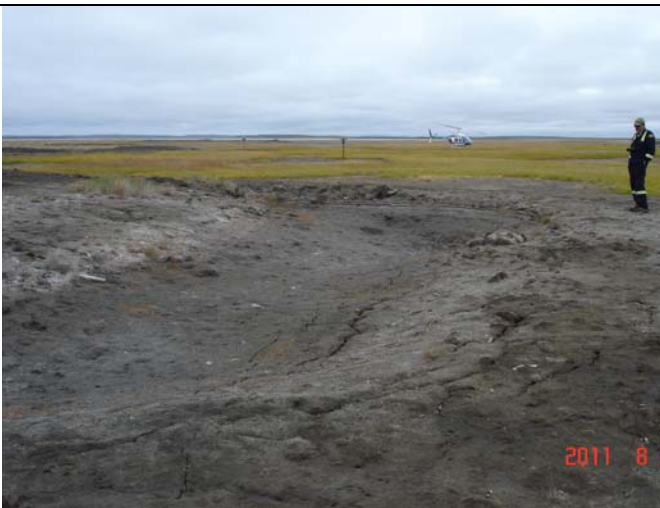
Figure 1 Aerial overview of drill sump, water ponding around the sump edges. Some subsidence on the sump cap, August 24, 2011.
