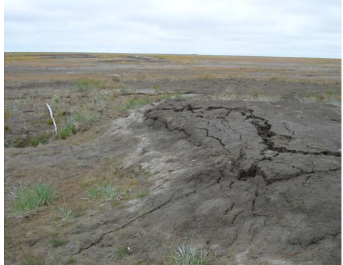
Figure 6 Camp sump south side subsidence and cracking, August 24, 2011.
