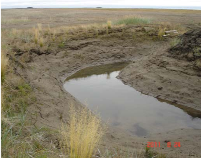
Figure 5 Camp sump with very deep north side subsidence and water ponding in the bottom, August 24, 2011.
