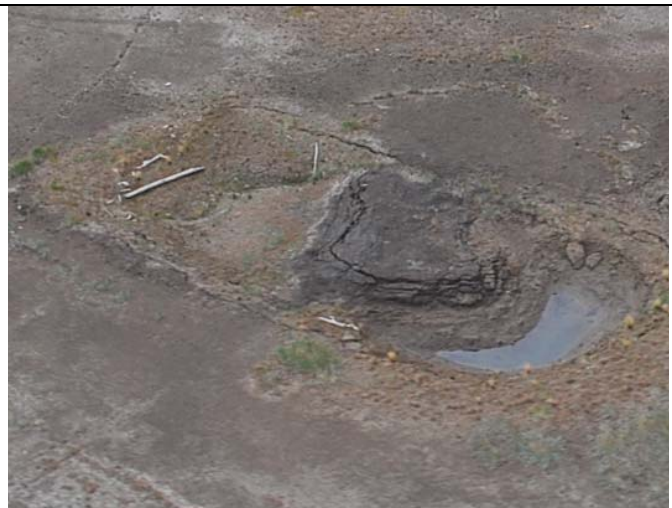
Figure 4 Aerial overview of camp sump. Large amount of deep subsidence and surficial cracking. Poor vegetation growth, coverage of ~15%, August 24, 2011.
