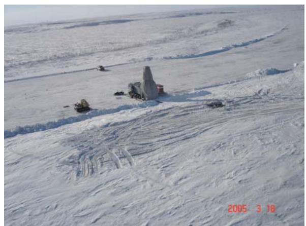
Figure 8. General. Drill at KP-T0 TPFSA.
