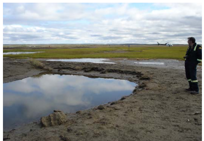
Figure 6 2002 Drill Sump subsidence at southend.
