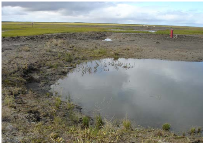
Figure 5 2002 Camp Sump subsidence at southend.
