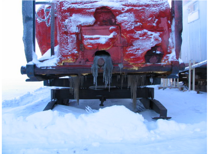
Figure 2. Sewage leaking from the sewage tank at the Grubens Sleigh Camp.
